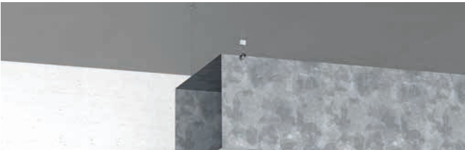
HVAC – rectangular duct
