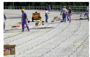
c) Repair and reinforcement of a bridge deck
