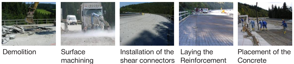
Figure 5 Simplified overview of the execution steps of a construction measure with overlay
